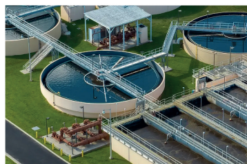
Water & Wastewater Treatment Plant
